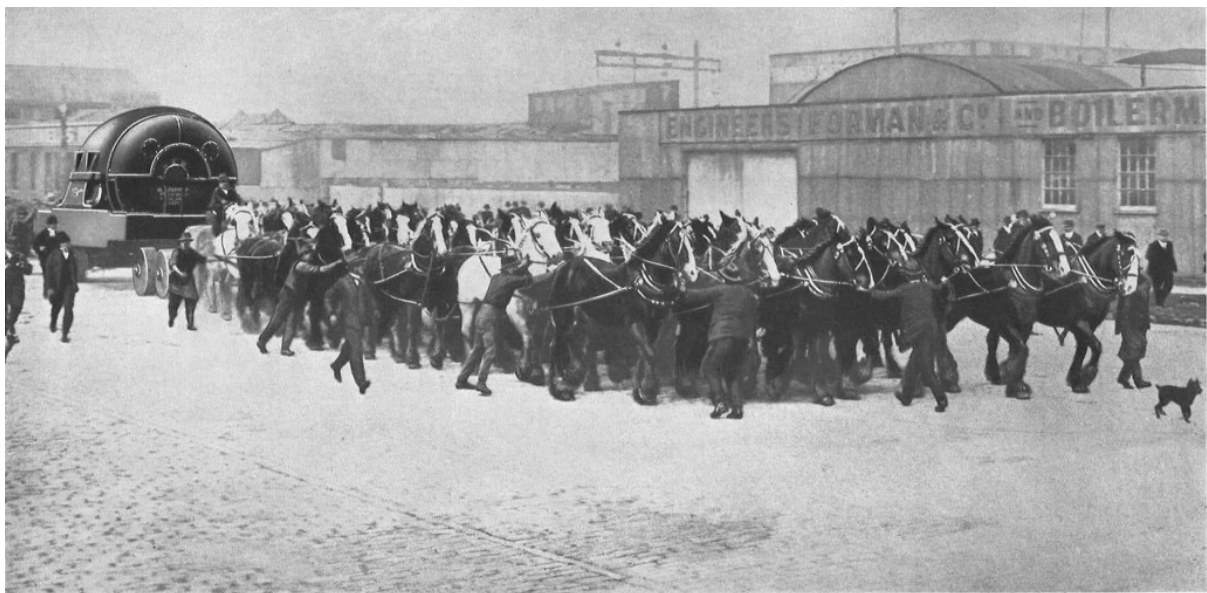
47-TON STATOR BEING CONVEYED THROUGH THE STREETS OF PORT MELBOURNE TO THE POWER STATION of the VICTORIAN RAILWAY COMMISSIONERS
